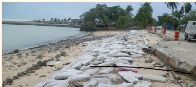
Damaged sea wall
