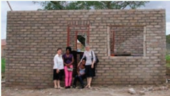
Land fencing and foundations
